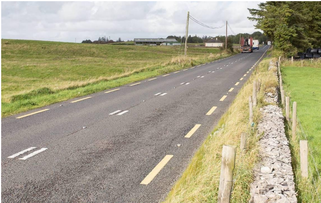
Plate 2.13 Existing N5 Road Pavement
